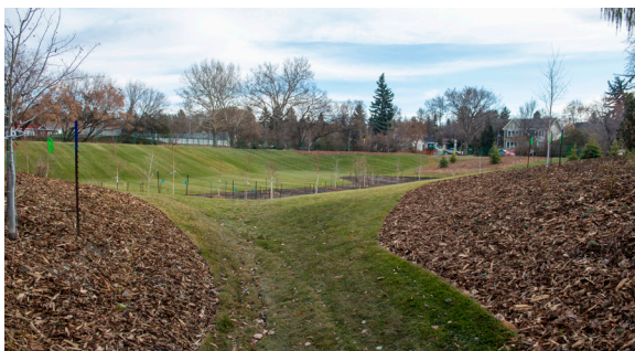
Dry ponds protect communities from flooding by slowing the entry of stormwater into the drainage system.
