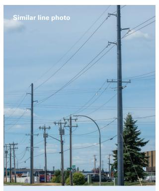
The poles for this project will look similar to the image above except they will have six wires on top (three on each side). Exact details may change based on finalized design.
