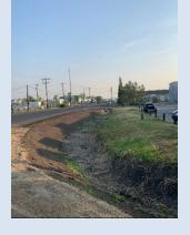
Majority of ditches were overgrown resulting in blocked flow paths. Vegetation was cleared and culverts repaired to increase flow capacities. New grass seed is being applied and will be maintained annually to maintain drainage functionality
