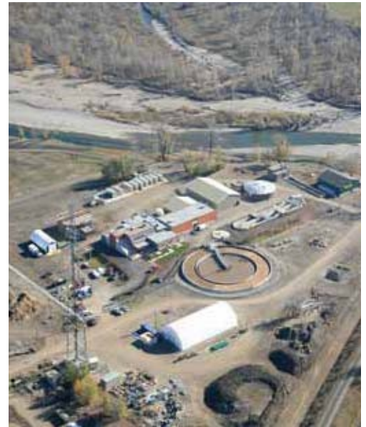
WWTP aerial photo
