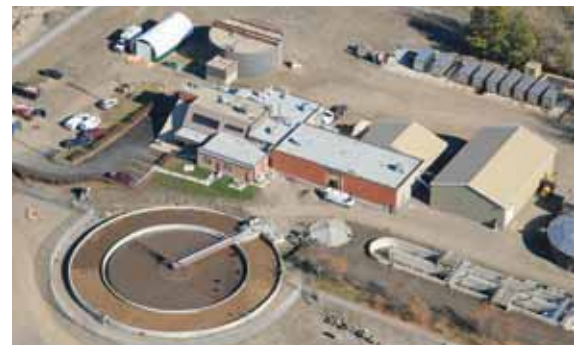
WWTP aerial photo
