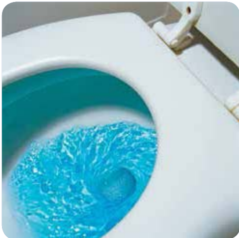
Blue dye tablets can be used to test for toilet leaks.
