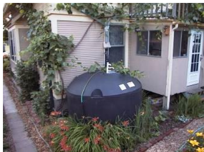
Residential rain barrel to harvest roof runoff for irrigating plants.
