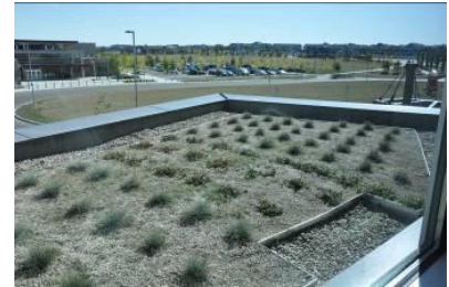
Newly planted green roof at Terwillegar Recreation Centre showing perimeter drainage, Edmonton, AB
