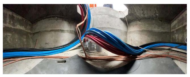
All cables installed within the base shall be layered from top to bottom in the following order: blue, black, red, white.
