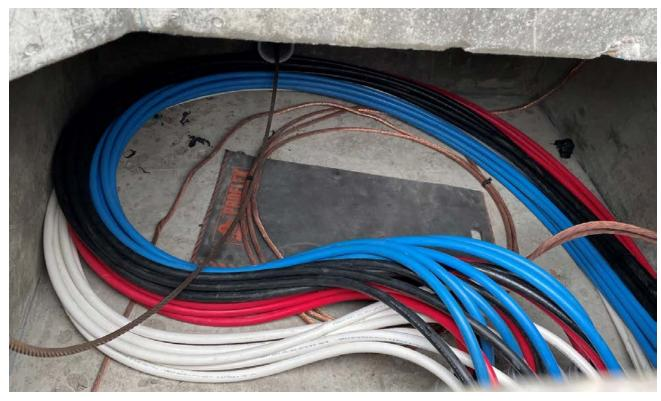
All cables installed within the base shall be layered from top to bottom in the following order: blue, black, red, white.
