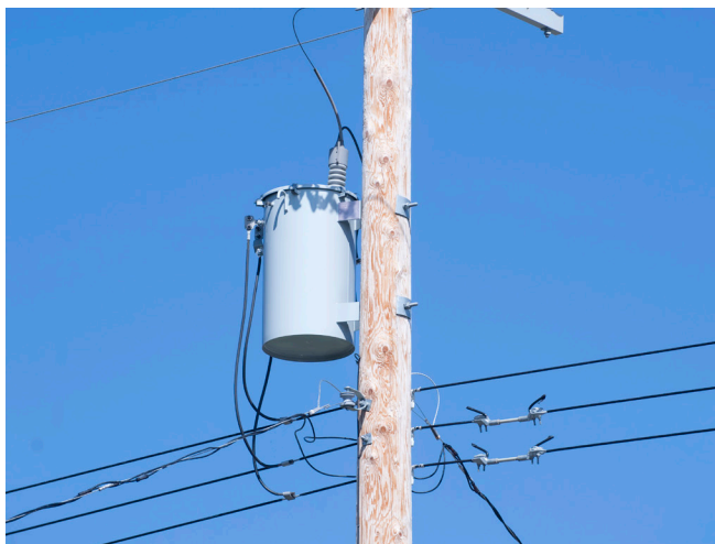
PCBs in electrical equipment are found in transformers such as this one, in the form of insulating oily liquid.
