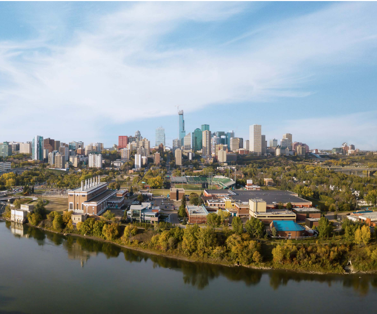
Rossdale Water Treatment Plant, Edmonton, Alberta, Canada
