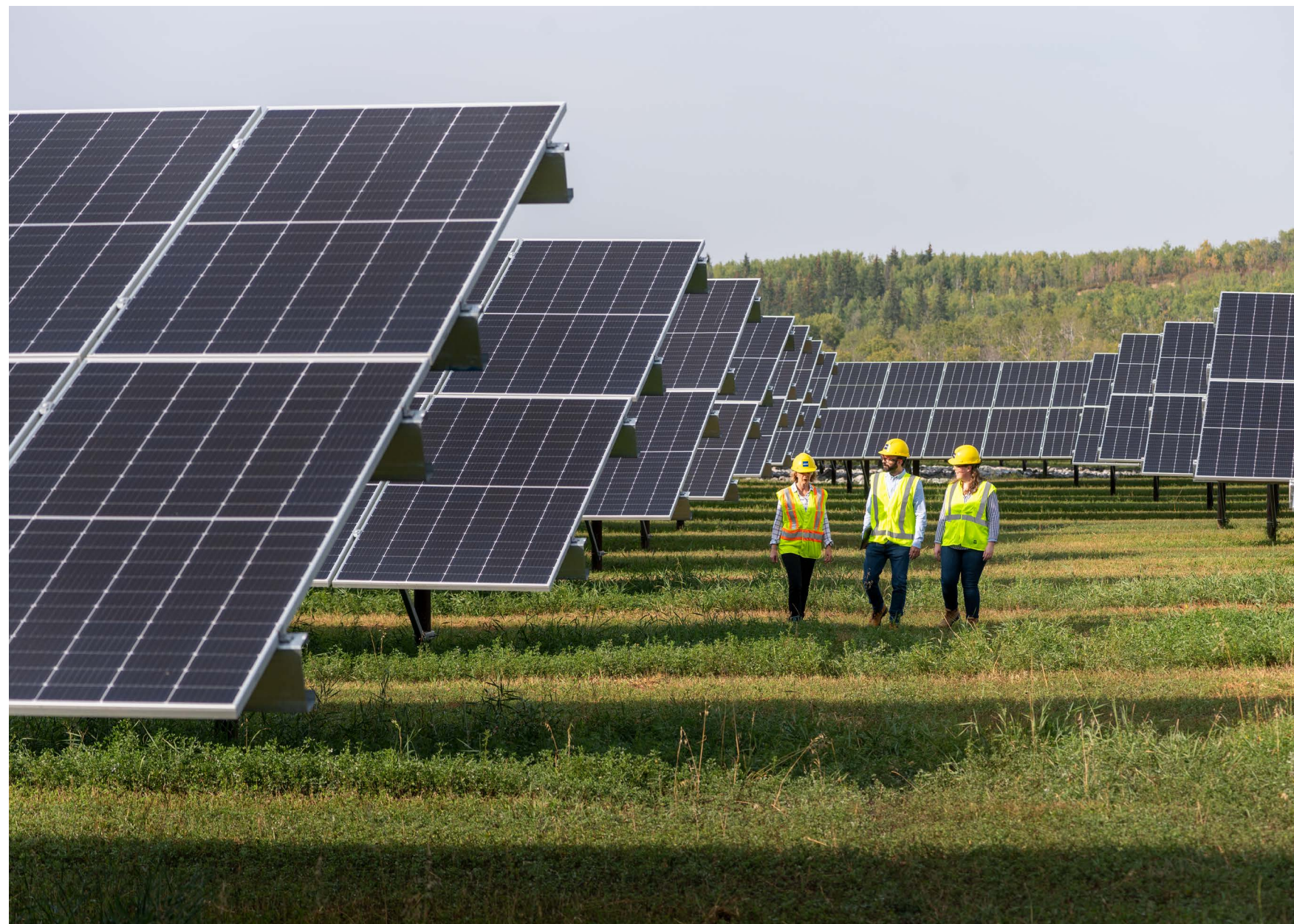
kísikāw pīsīm Solar Farm, Edmonton, Alberta, Canada
