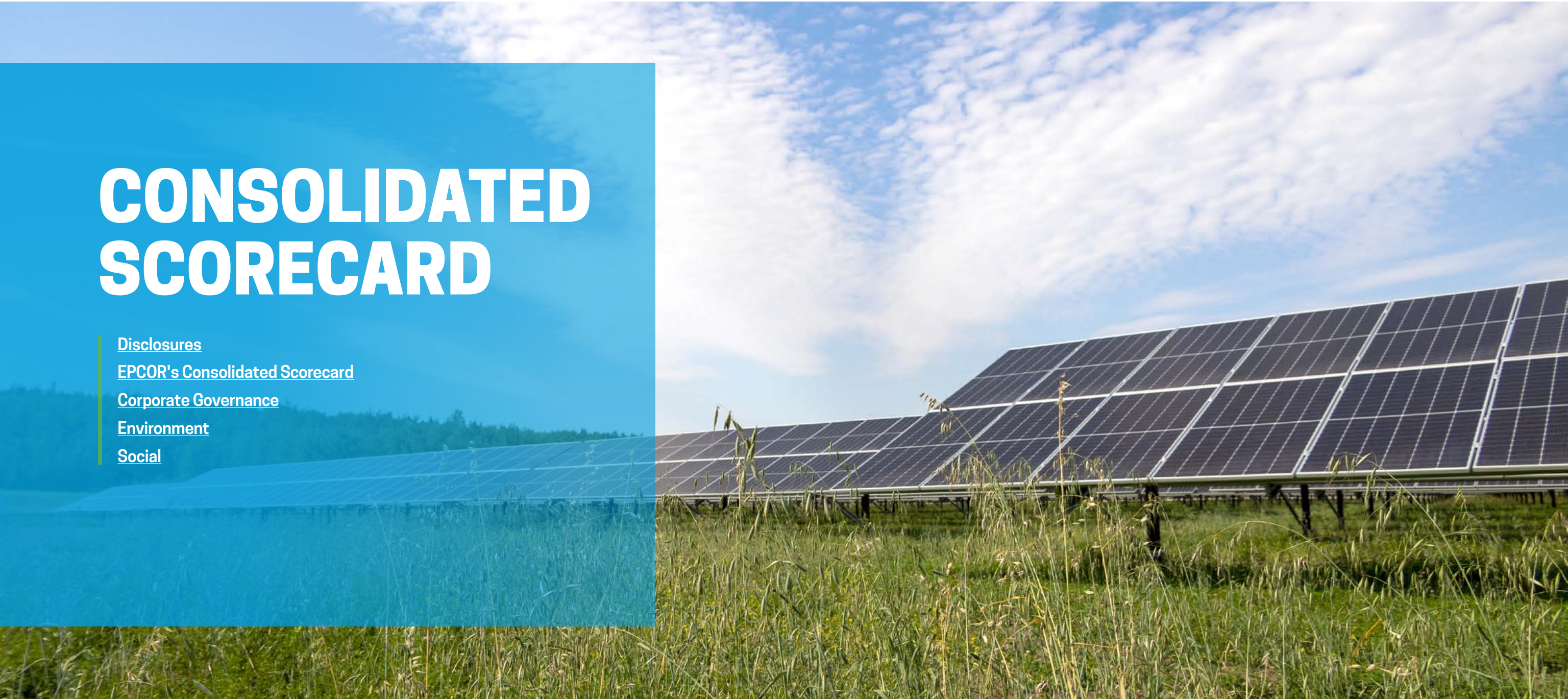
E.L. Smith Water Treatment Plant, kisikaw-pisim solar farm, Edmonton, Alberta, Canada
