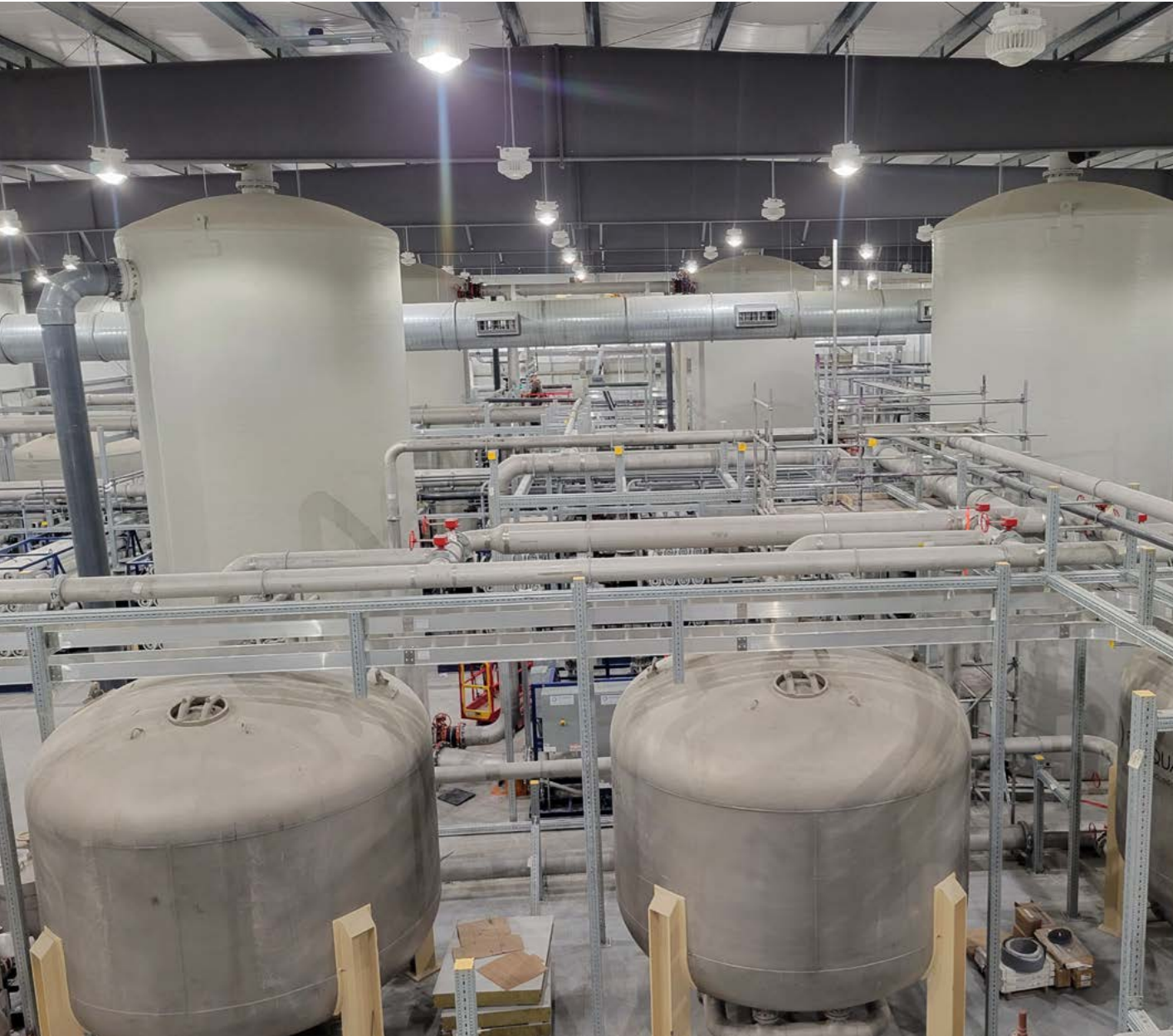
EPCOR's Water Treatment Plant, Darlington, Ontario, Canada
