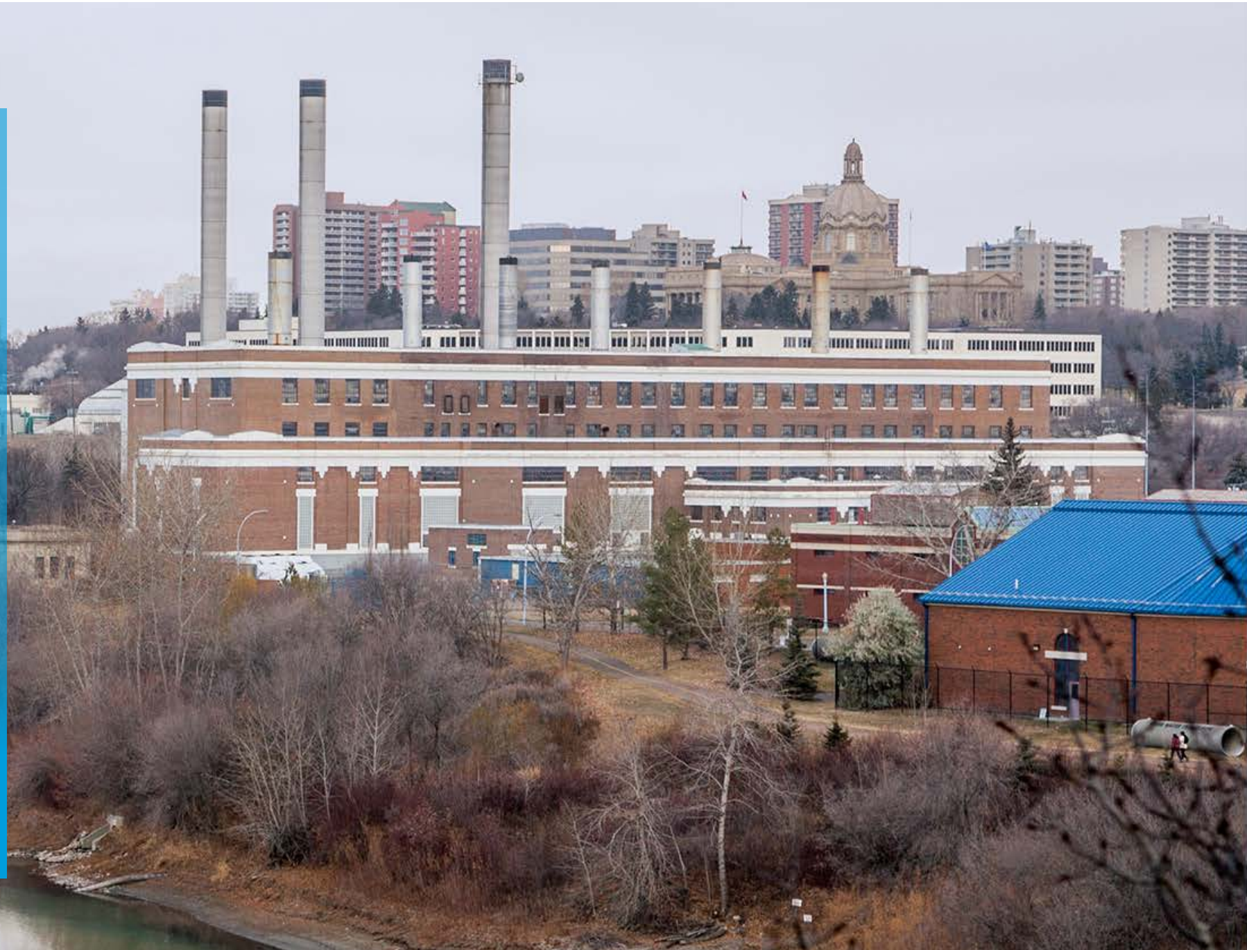
Rossdale Water Treatment Plant, Edmonton, Alberta, Canada
