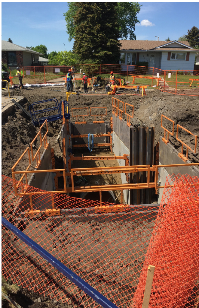
Open-Trench Construction
