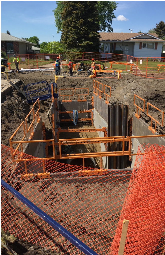
Open-Trench Construction
