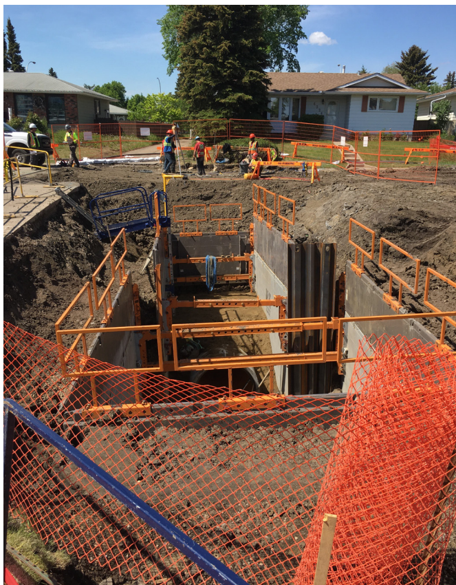
Open-Trench Construction
