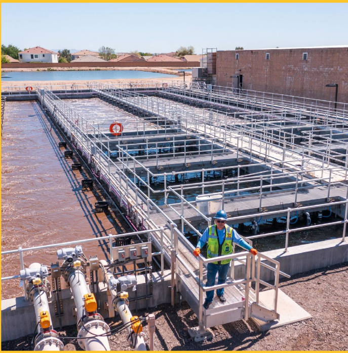
Upgrades at the Pecan Water Reclamation Facility, AZ, were completed in 2022.
