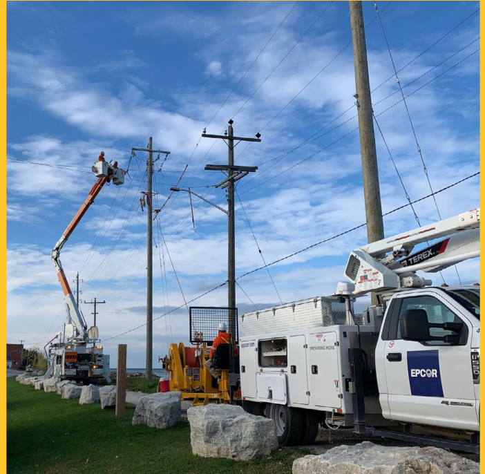
A crew completing a pole line rebuild in Collingwood, ON.
