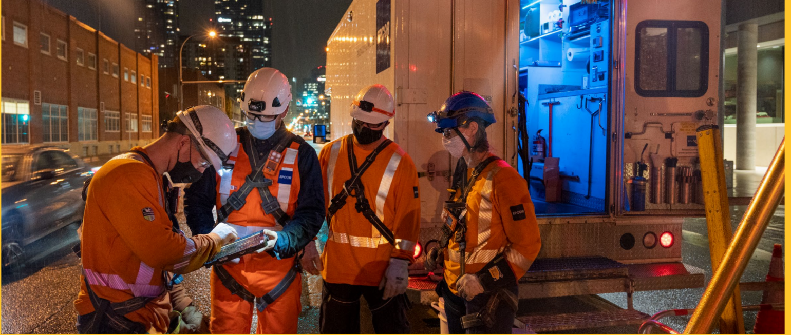
An electricity underground crew in Edmonton, AB.
