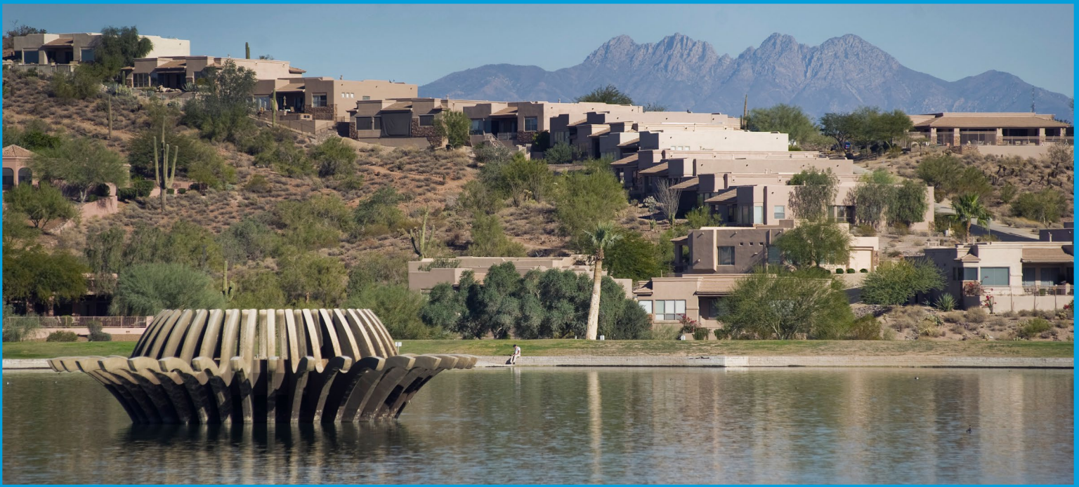
EPCOR supplies Fountain Hills, Arizona, with potable water.
