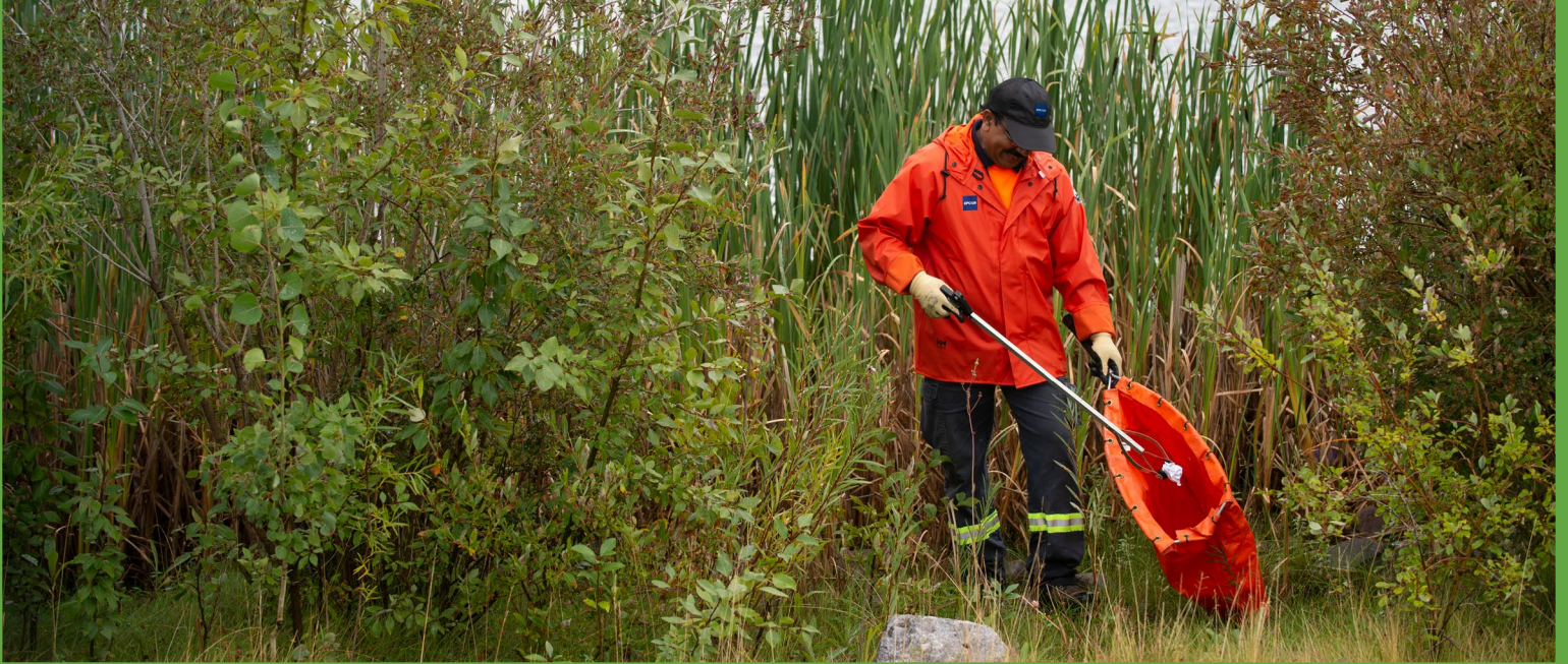
Maintaining the Brintnell Stormwater Facility in Edmonton, AB.
